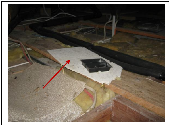
Photograph 2: Unit 1 store ceiling space – sheet debris (refer sample 5684 – A2) No Asbestos Detected
