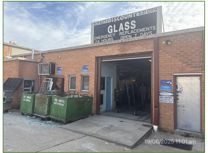
Rear of the Units
